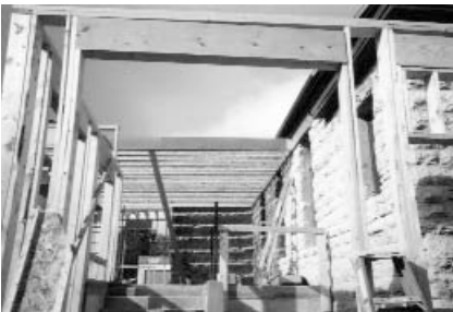
Construction photos: Harold Kost, Jamesport MO
